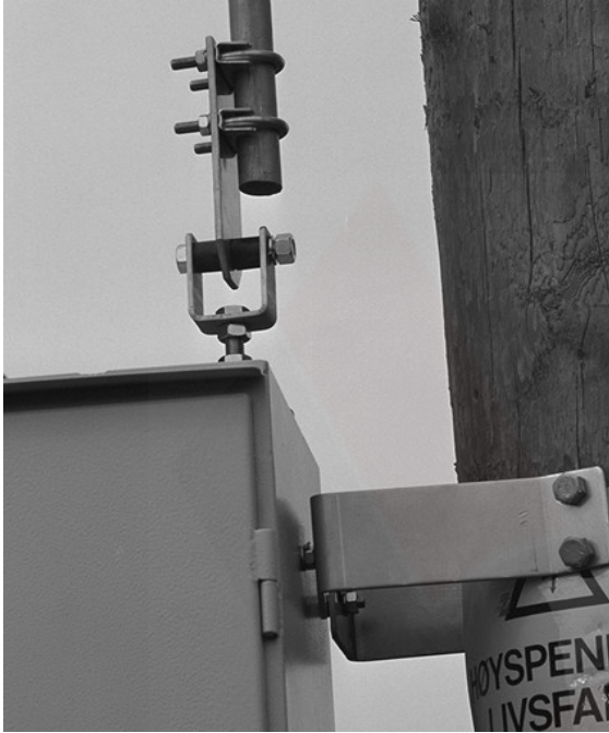
Exterior detail, showing the adaptor for maneuvering rod attachment and bracket for wooden pole.
