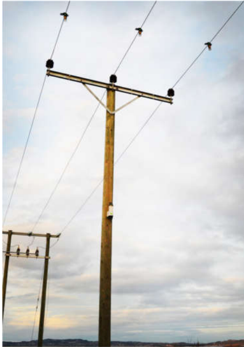
Parallel feeders or multiple feeders in the same pole
